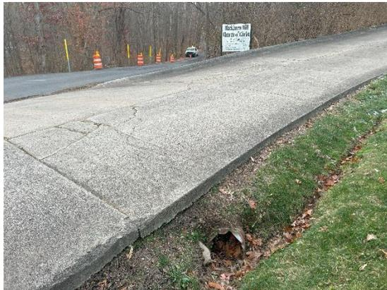
site on the north end with no evidence of recent flow of water. We could not find any inlets in the ditch on the west side of the roadway within the project area. A cross pipe was observed going underneath the concrete driveway; however, we could not find an outlet on the west side of Blackburn Road. Due to the condition of visible storm drains and some inlets/outlets not being visible, we recommend a private utility locator be engaged to map the storm drains in the area and use camera video
